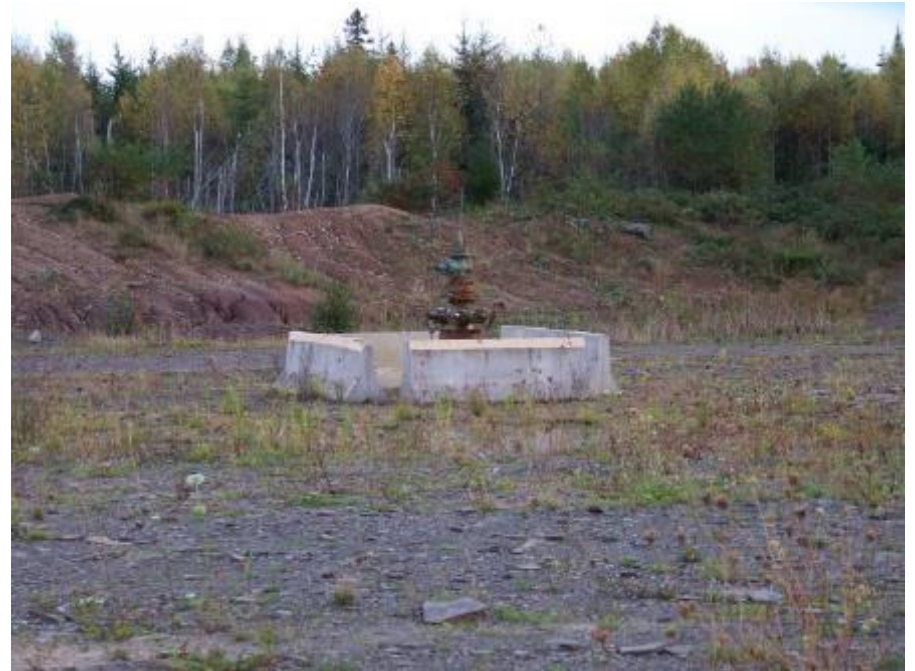
Abandoned well before reclamation processes Hants County, Nova Scotia Source: Halifax Media Co-op, June 2014
