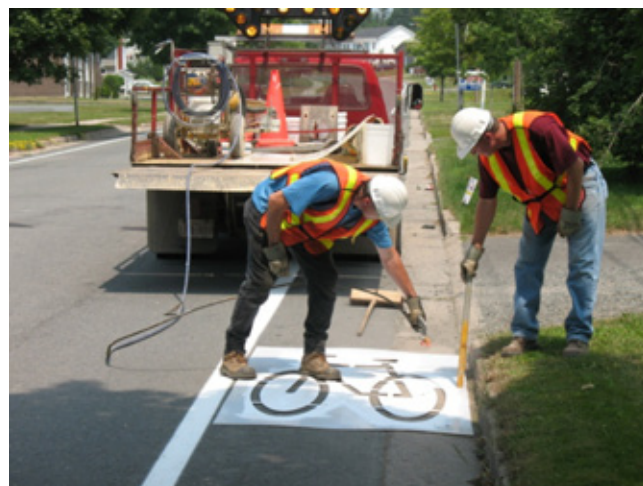
Figure 5.12: Pavement Signage on Paved Shoulder
