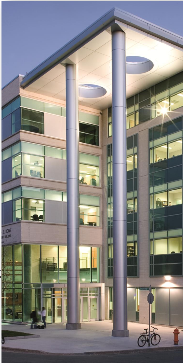
General Contractor: Pomerleau / Photographer: Janet Kimber
