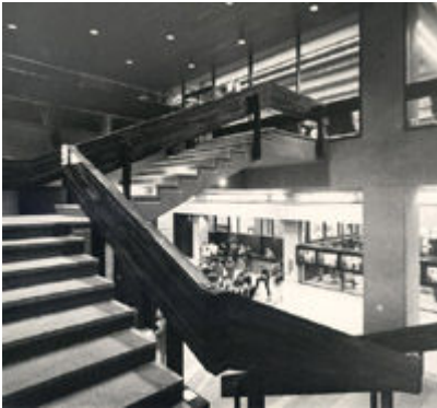
Killam Memorial Library - Interior - Staircase, n.d.
