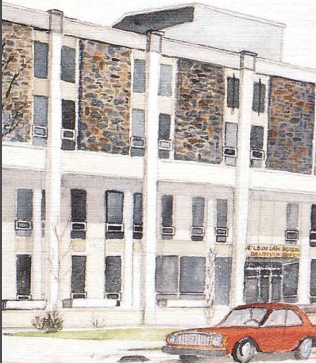
WELDON BUILDING 1987 - PRESENT (POST-FIRE)
