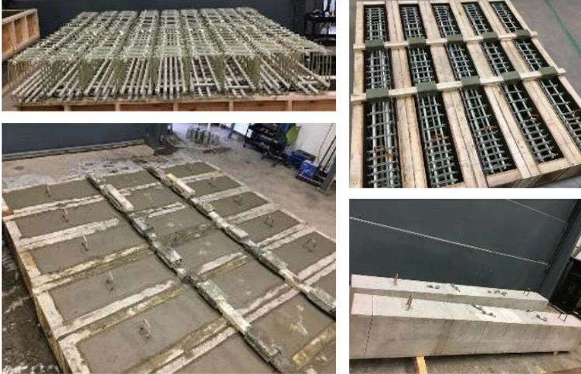
Figure 5. GFRP-reinforced concrete beam fabrication
