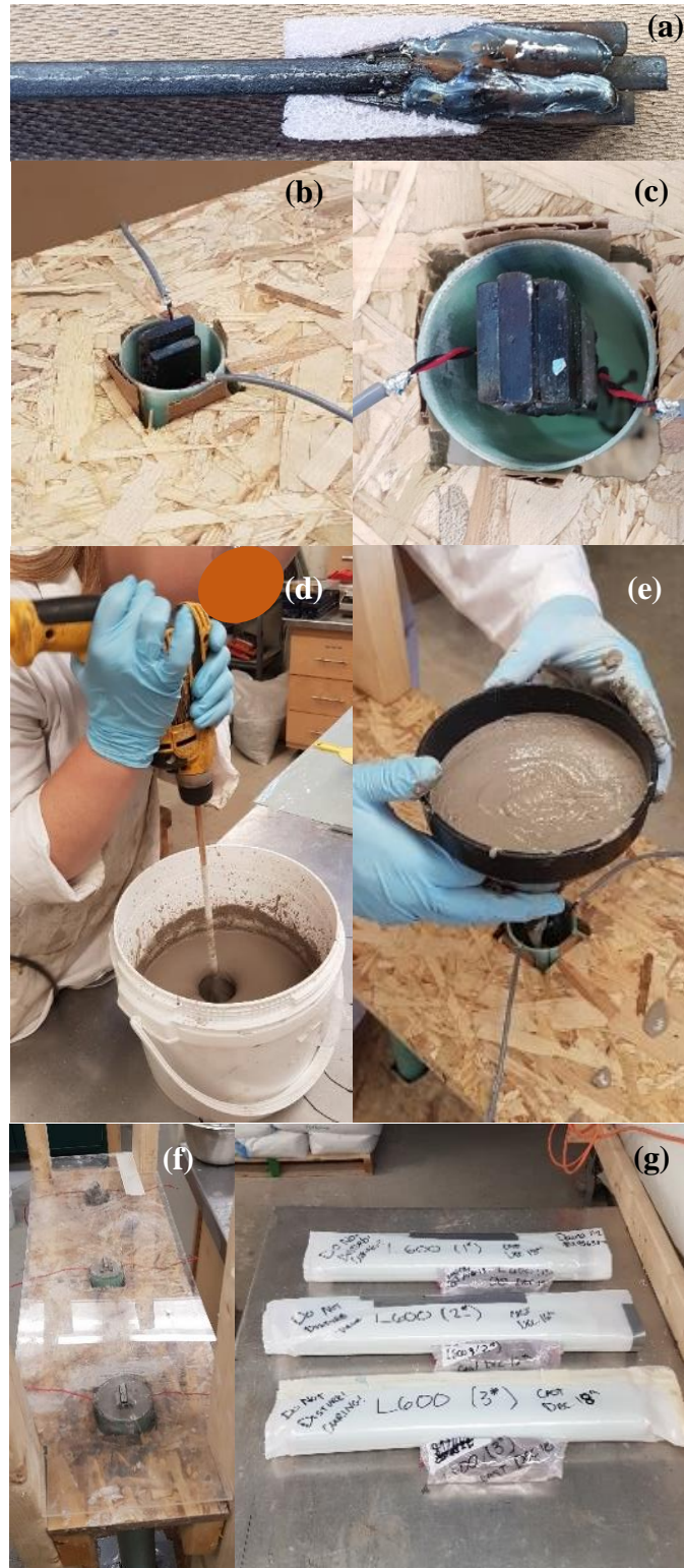
Fig. 3. Specimen fabrication: (a) steel core is prepped with tabs and expanded polystyrene (b) and (c) tube is shimmed to ensure steel core and FRP tube are aligned; (d) self-consolidating grout is mixed; (e) grout is funneled into FRP tube; (f) fiberglass cover is placed; (g) specimens cured in plastic bags at room temperature.
