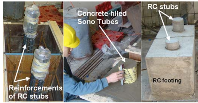
Fig. 3. Preparation of RC footings and stubs
