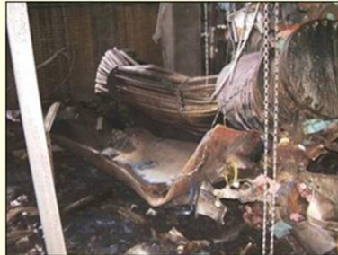
Heat Exchanger Rupture
