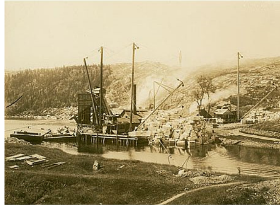
Historic granite quarry at Purcell's Cove (PANS)
