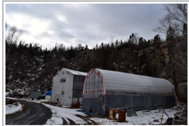
Figure 14. View of Purcell's Cove Quarry today.
