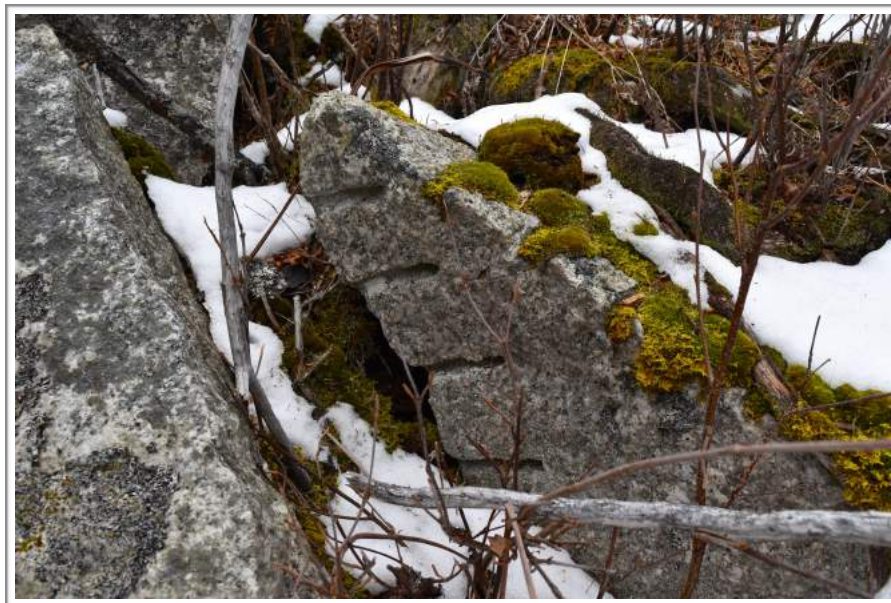
Figure 22. Series of wide holes indicative of blasting.
