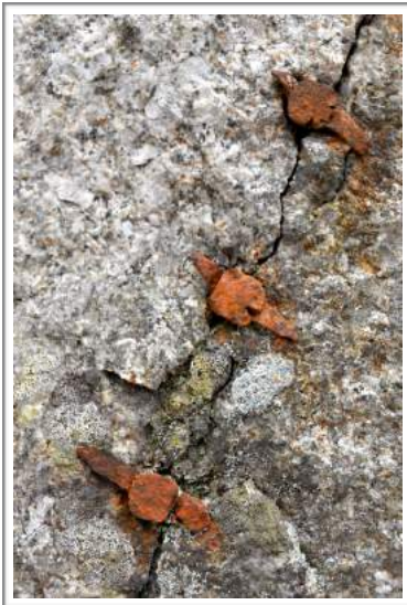
Figure 31. Shims and wedges at Purcell's Cove.
