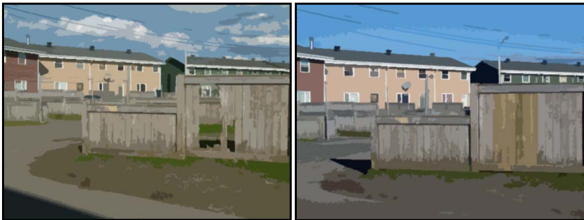
Encouraging Indicators: A vandalized fence is fixed between site visits
