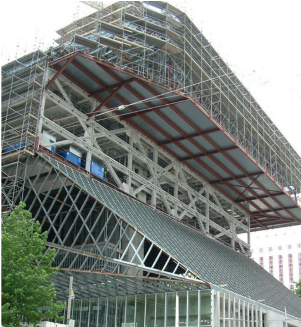
OMA, Seattle Public Library, Seattle, WA, 2004. Construction photo.
