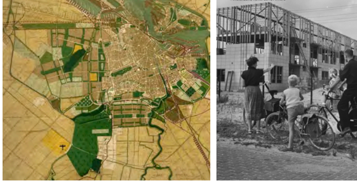
(lft) Green Plan Amsterdam (AUP 1934); (rt) Photograph of housing construction 1952, Slotemeer, Amsterdam Nieuw-West, using 'Airey' technique, City Archives.
