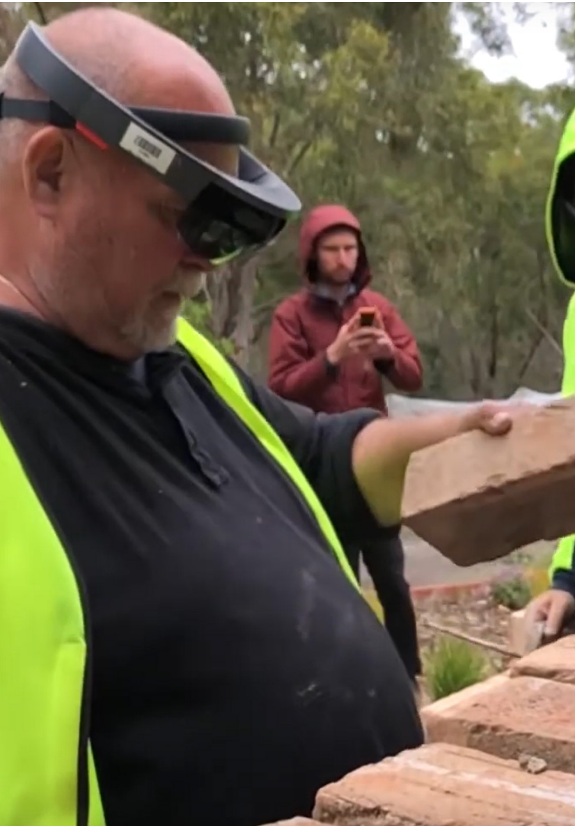
Fologram, bricklaying with augmented reality.
