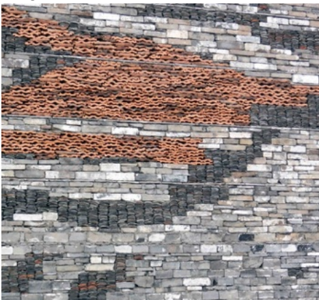
Wang Shu, wall detail
