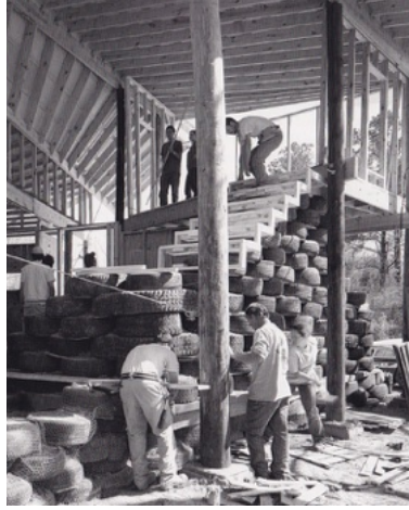
Students building Shiles House, Rural Studio
