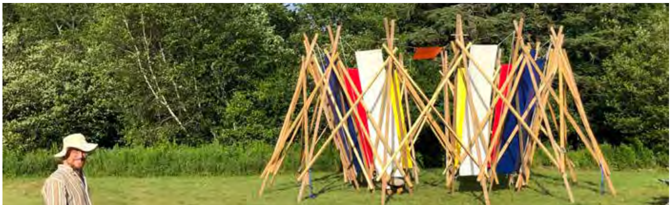
View of temporary structure installed on course build site (summer 2023). In view, collaborator Mark MacKinnon
