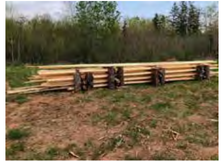
Framing materials harvested and ready for assembly on site in Millbrook First Nation. See: community website
