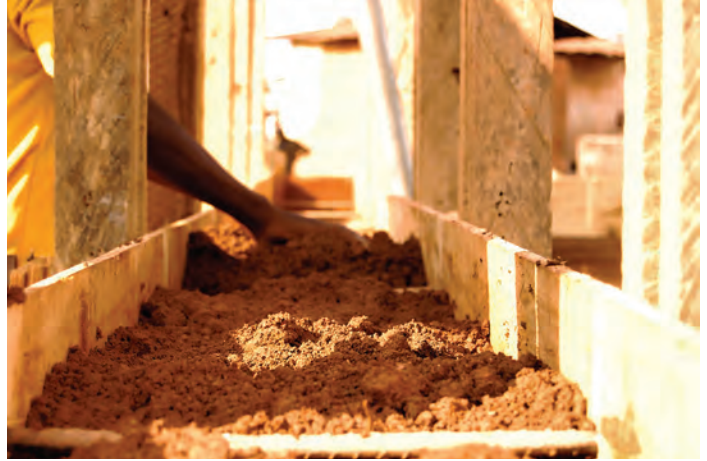
Rammed Earth Formwork, Ghana, Solterre Design.
