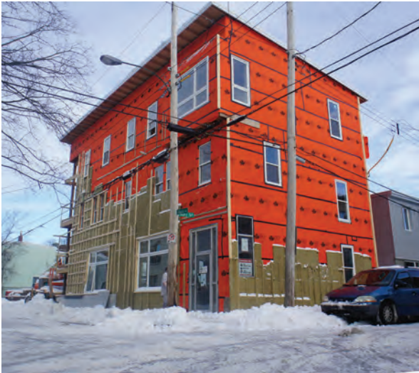
Air Barrier and Insulation Installation, EAC Offices, Solterre Design.
