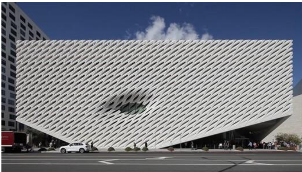
Façade design of The Broad in Los Angeles, showing a pattern of mass-customized fibre-reinforced concrete panels which create a “veil” shading the interior spaces of the museum. Designed by Diller Scofidio + Renfro, image via Archdaily 2015.
