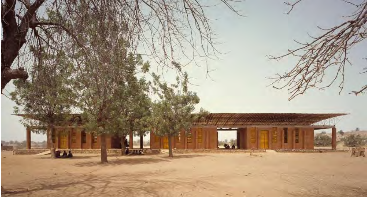
^ Primary School, Gando, Burkina Faso, Francis Kéré, 2001.
