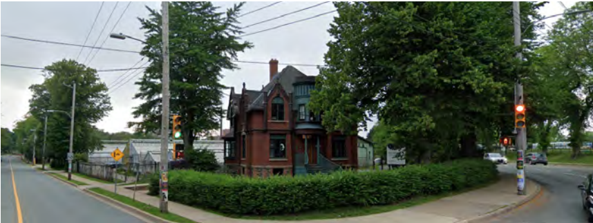
POWER HOUSE AT BELL RD/SACKVILLE INTERSECTION
