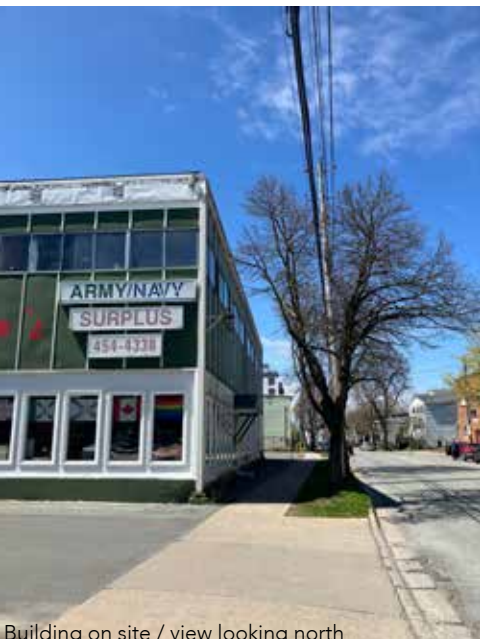
Building on site / view looking north
