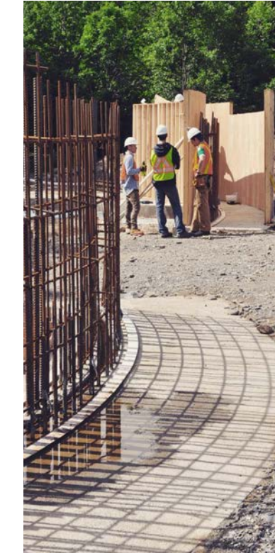
Highlands Gridshell Cheticamp, Cape Breton, NS Design-Build Project (2016)
