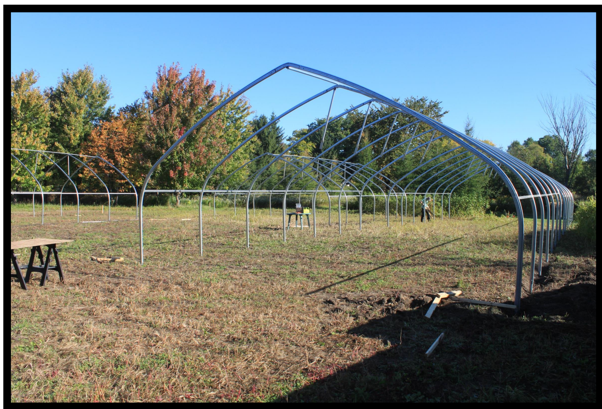
Fig. 1. High tunnels are under construction.
