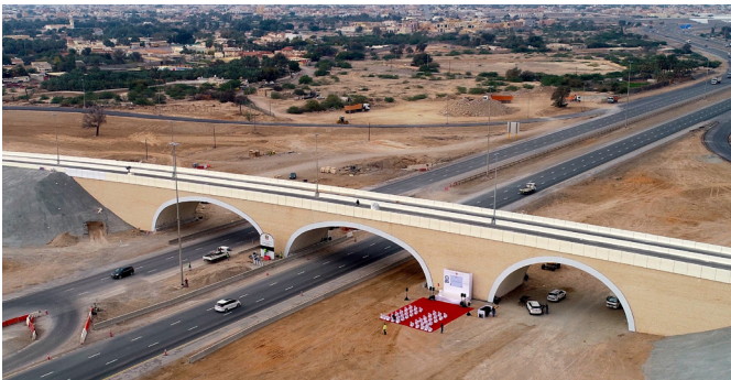
▲ The Faculty of Engineering's focus on helping companies develop innovative products has led to a Guinness book of world record. The Shammal Bridge near Dubai, United Arab Emirates (UAE), was recently named the world's largest metal buried bridge with a span of 32.39 m. The project uses Atlantic Industries Limited new Ultra-Cor engineered structural steel plate developed in Dalhousie's Heavy Structures Lab.
