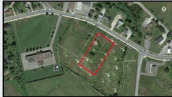
Aerial View of Property Including Optimum Building Layout
