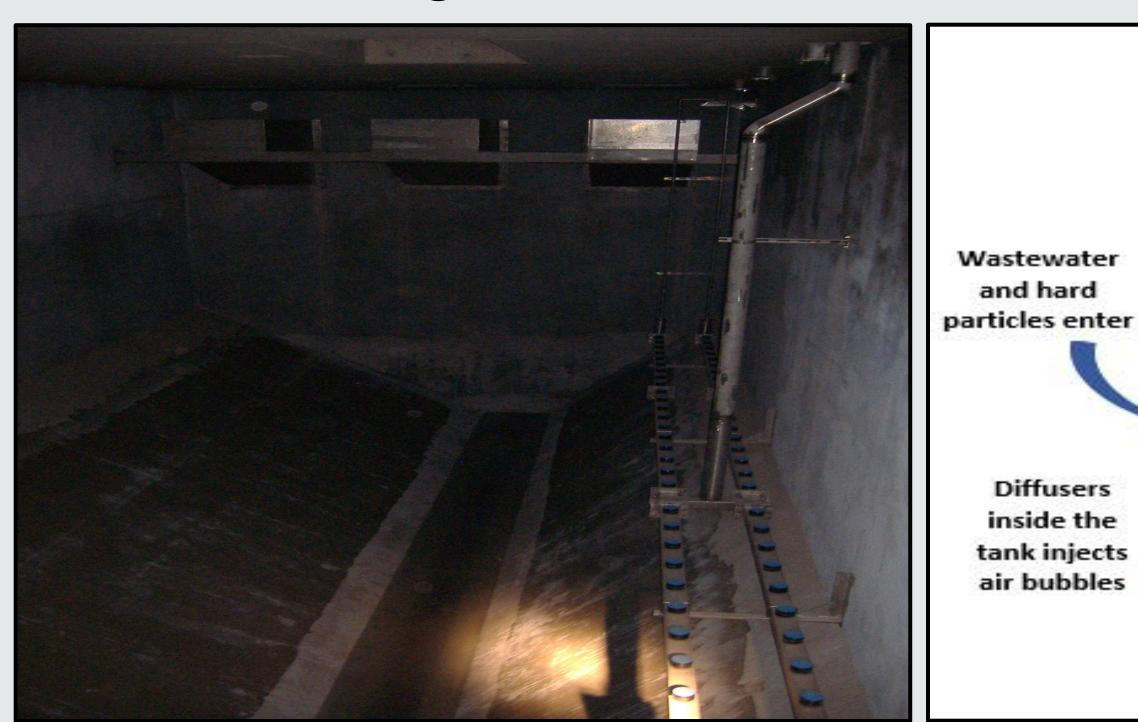
Inside the grit (hard particle) removal system is shown to the above left with air diffusers seen in two rows on right side. The injection of air reduces the density of the fluid inside the tank facilitating heavier particles to fall to the bottom. In order to determine efficiencies of particle removal, various flow rates and grit quantities would need to be tested. The right photo is a complete model with all inputs and outputs.
