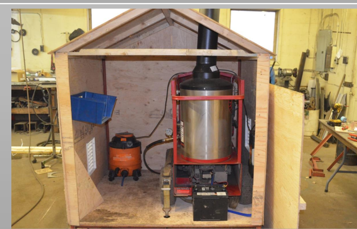
Stage 2: Equipment & Electrical
