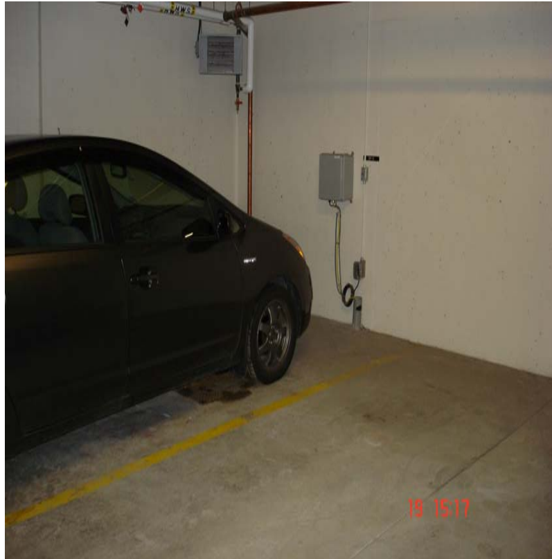
Photo Numbers: 2013 - 06 - 19 (1517) Pit is under right front Tire.
