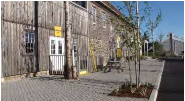
Fig.2 Permeable Paving Example on Hawthorne Street, Yarmouth NS
