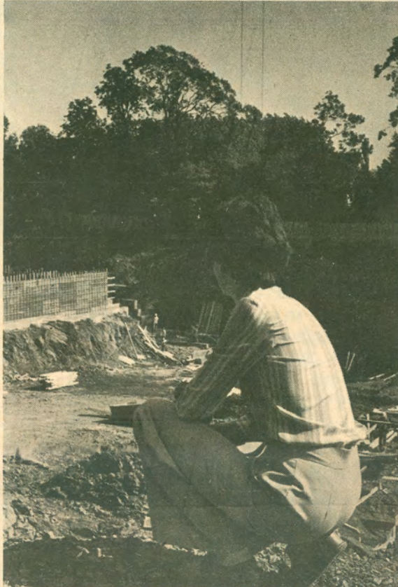
Information Office staffer Kate Carmichael surveys the progress on the Physical Education, Recreation and Athletic Centre, progress that university planner Jim Sykes says is "pulsing ahead" toward the late-1978 completion target.
