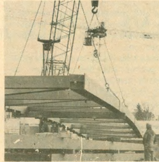
4 By January, 1978, the huge trestles which support the fieldhouse floor had arrived and were being put in place. This was a major step in the construction of the complex.
