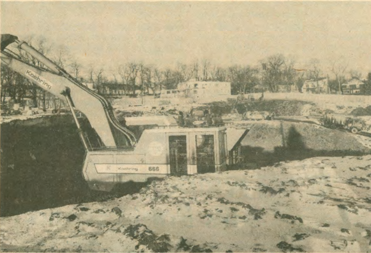
2 By December, 1976, the hole in the ground took shape.
