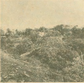
1 The first trees were cut on Oct. 14, 1976.
