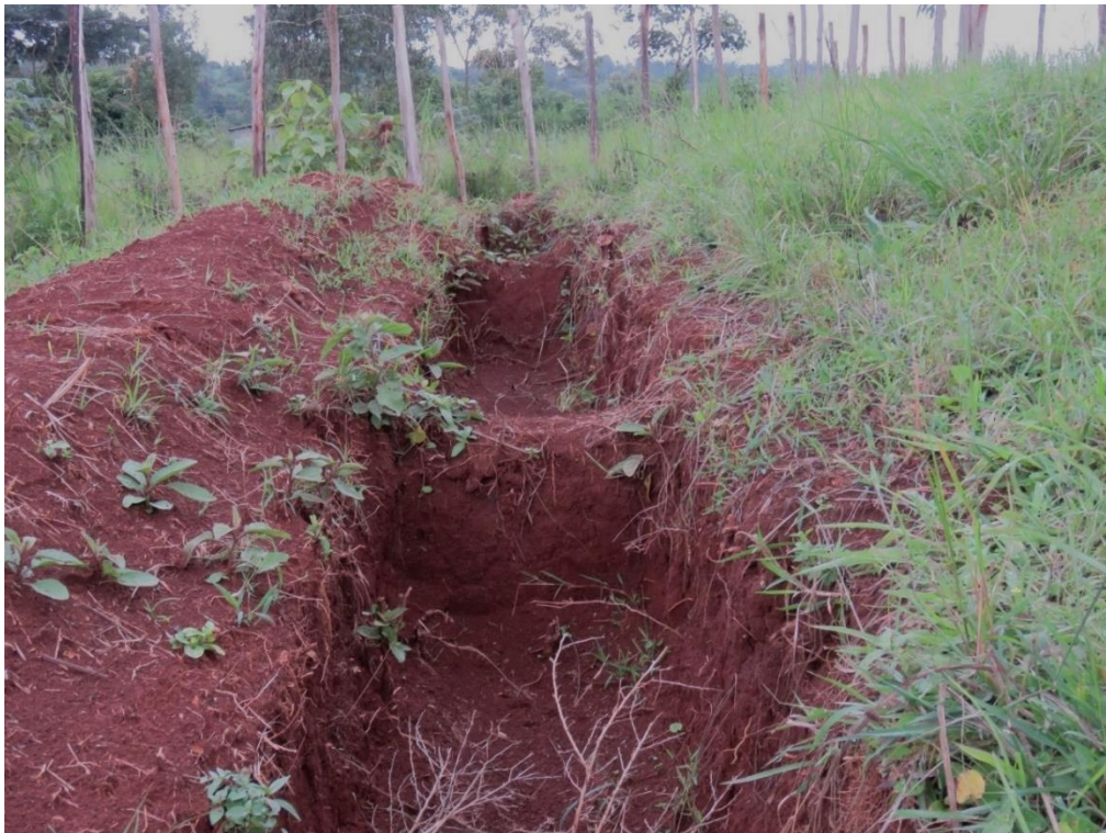
Figure 6: Soil erosion prevention method, as constructed by students during training
