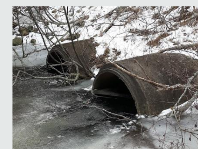
Above: circular culvert.
