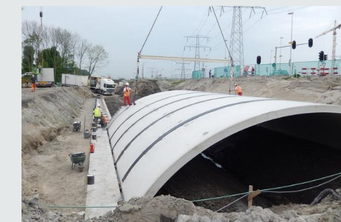
Above: Arch culvert.
