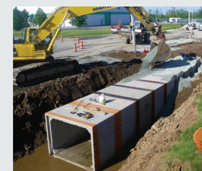
Above: Box culvert.
