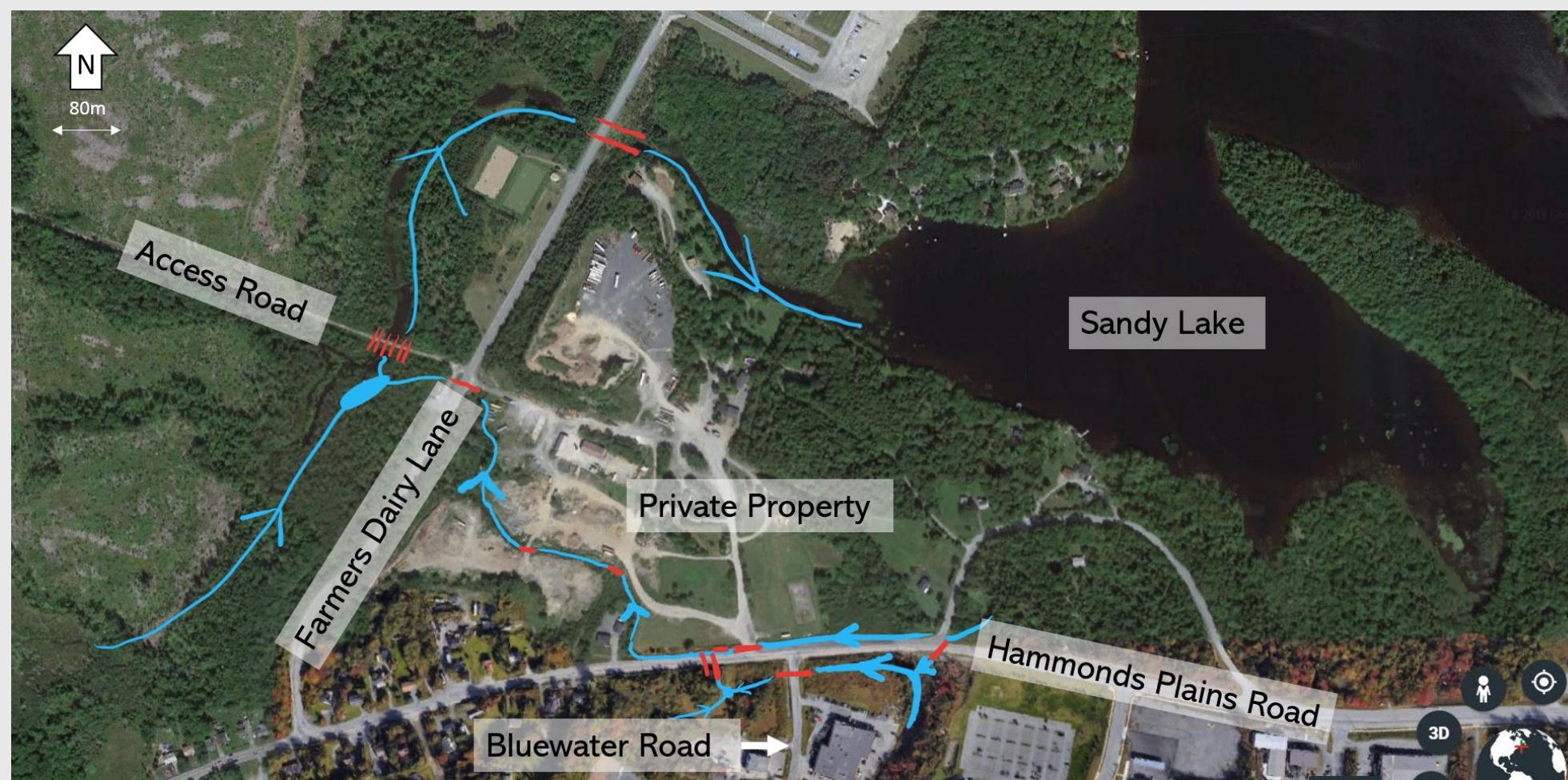
Above: Existing channel and project site. Hammonds Plains, Nova Scotia.
